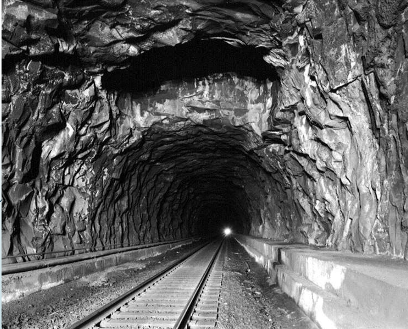
Bergen hill tunnel: source – Google images : horse shoe shaped tunnel
