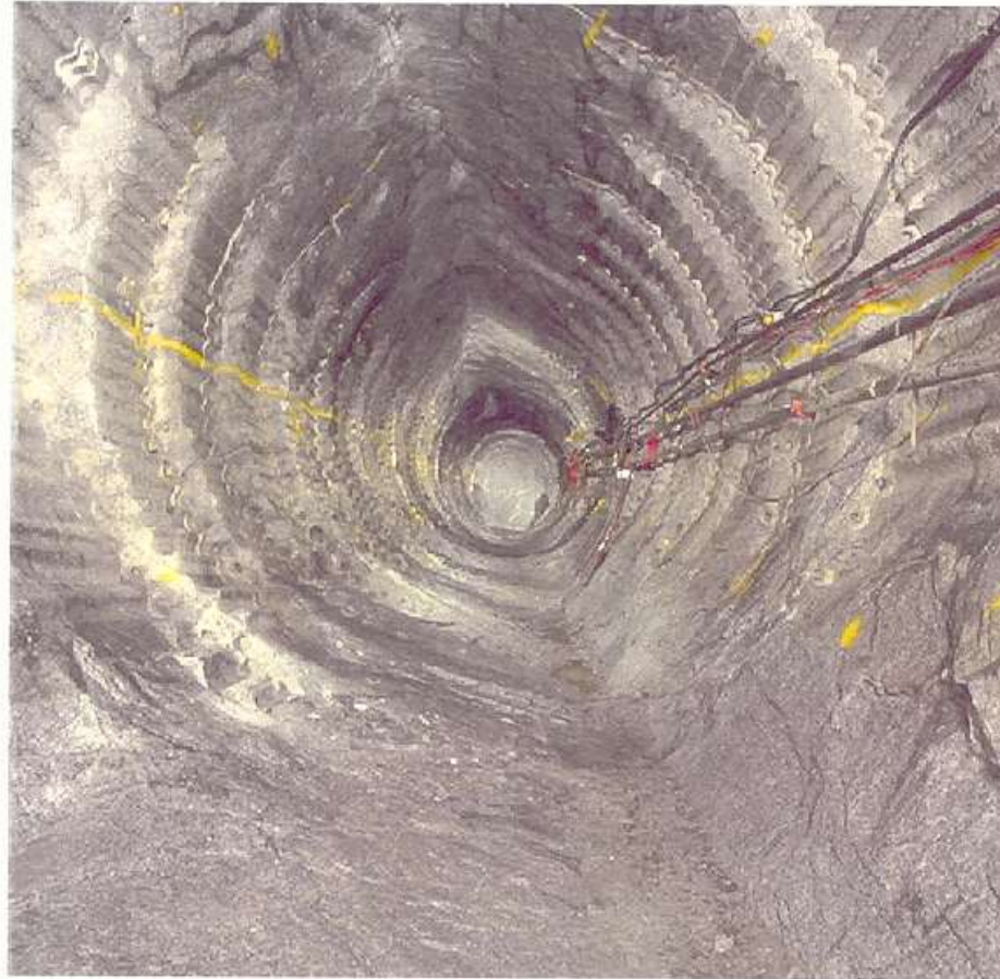
Mine-by Experiment Tunnel Showing Development of V-shaped Notches in the Roof and Floor of the Tunnel
