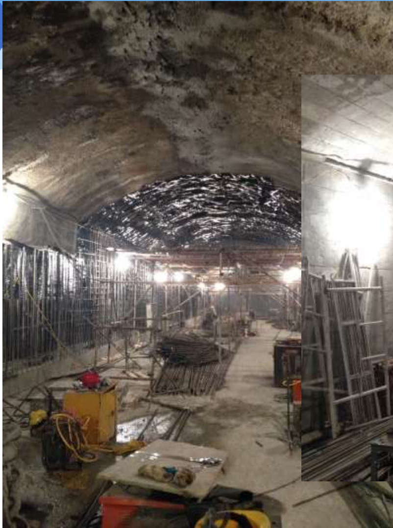
The steel support dismantlement
