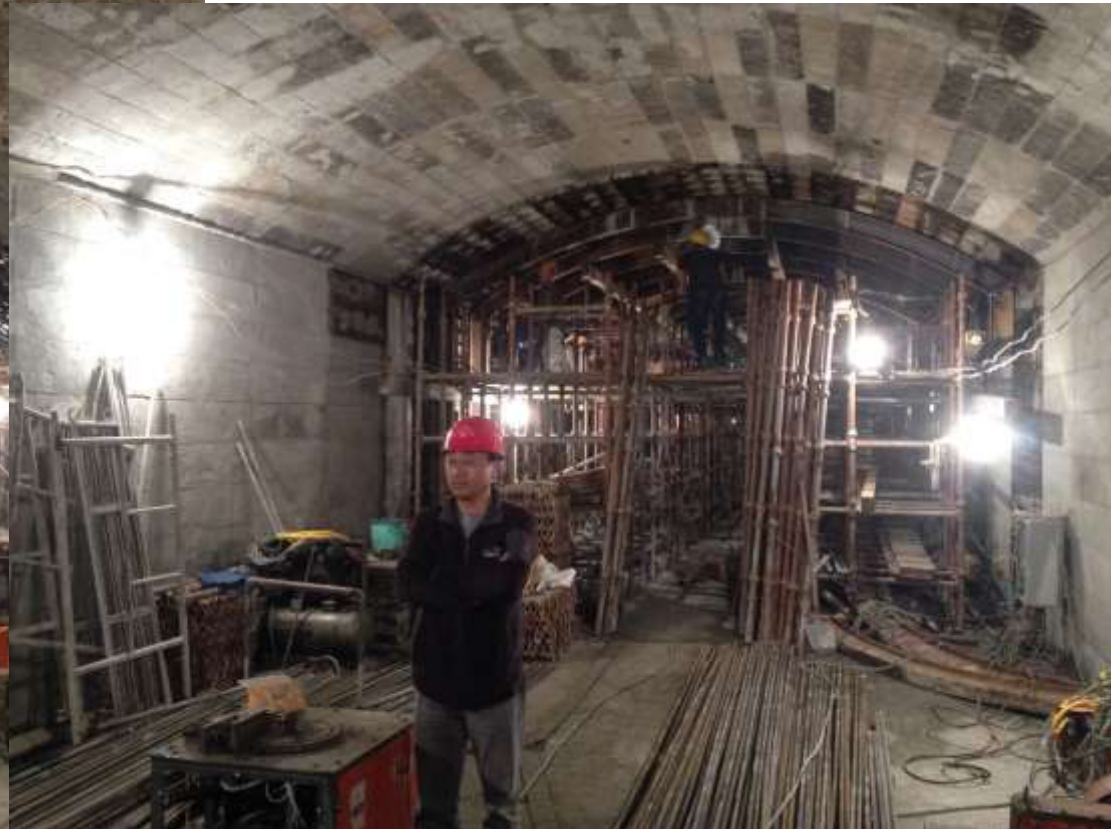
The secondary lining construction
