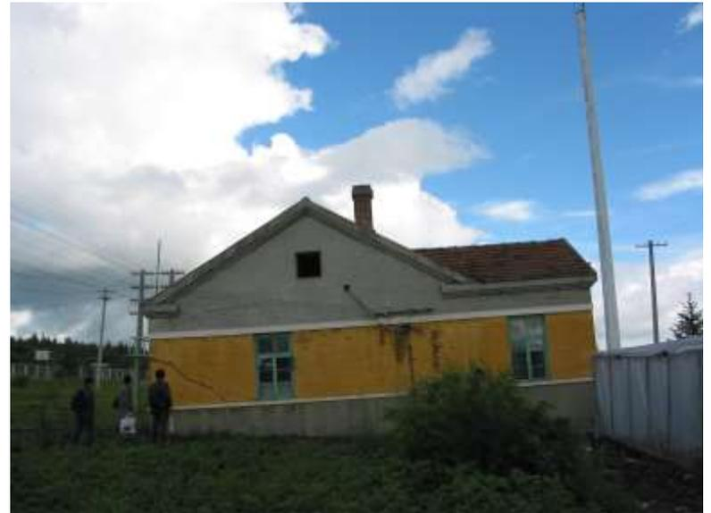
Damages related to thaw settlement due to thawing of ice-rich permafrost
