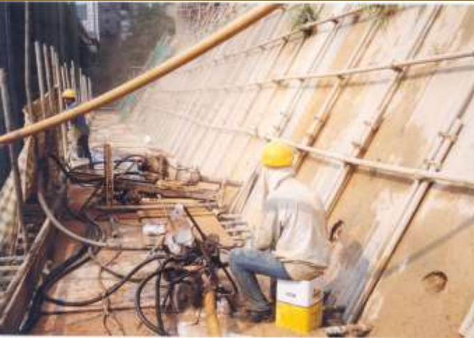
Pneumatic Drilling
