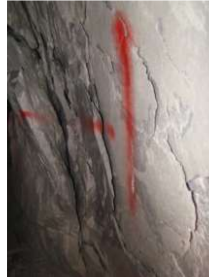
Test tunnel C
