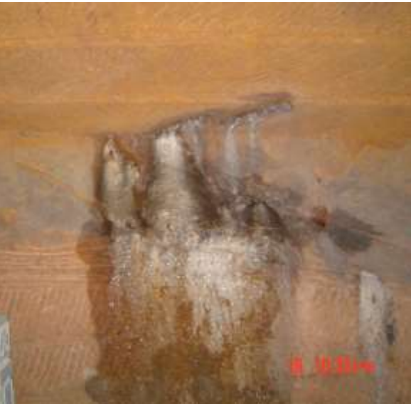
New calcareous sinter in new cracks
