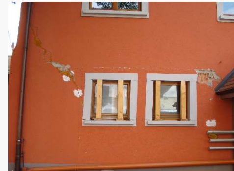
Ground Heave due to Conversion of Anhydrite to Gypsum
