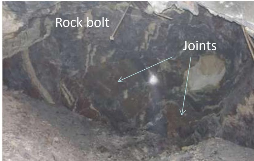
(1) Large scale collapse at roof in 3# Lab, 13 April, 2015, volume: 1000m<sup>3</sup>
