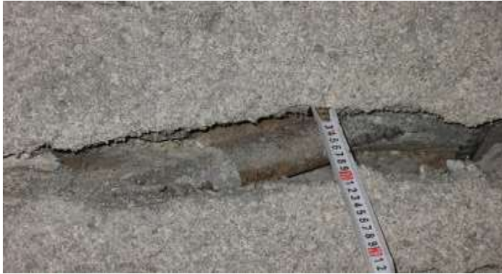
Shotcrete cracking and distorted steel bar at the downstream spandrel of the powerhouse
